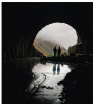
Kevin Muñoz Guillermo Gaviria Echeverri Tunnel Colombia.
